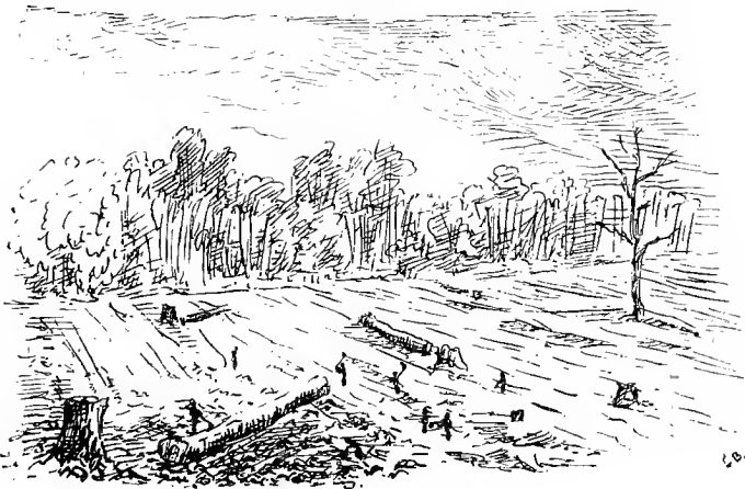
CLEARING THE GROUND.
